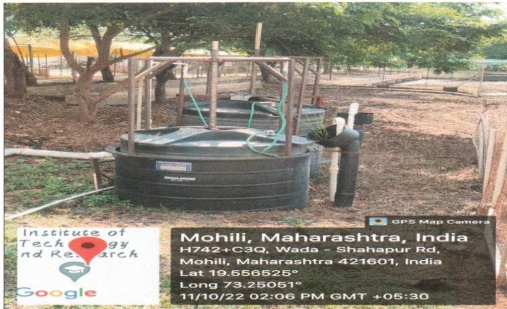
Biogas Plant near A wing building
